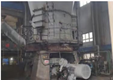
After Retrofit of the 1,250 kW Coal Pulverizers
