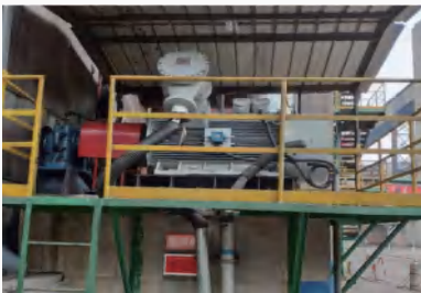
After Retrofit of the 900 kW Induced Draft Fan
